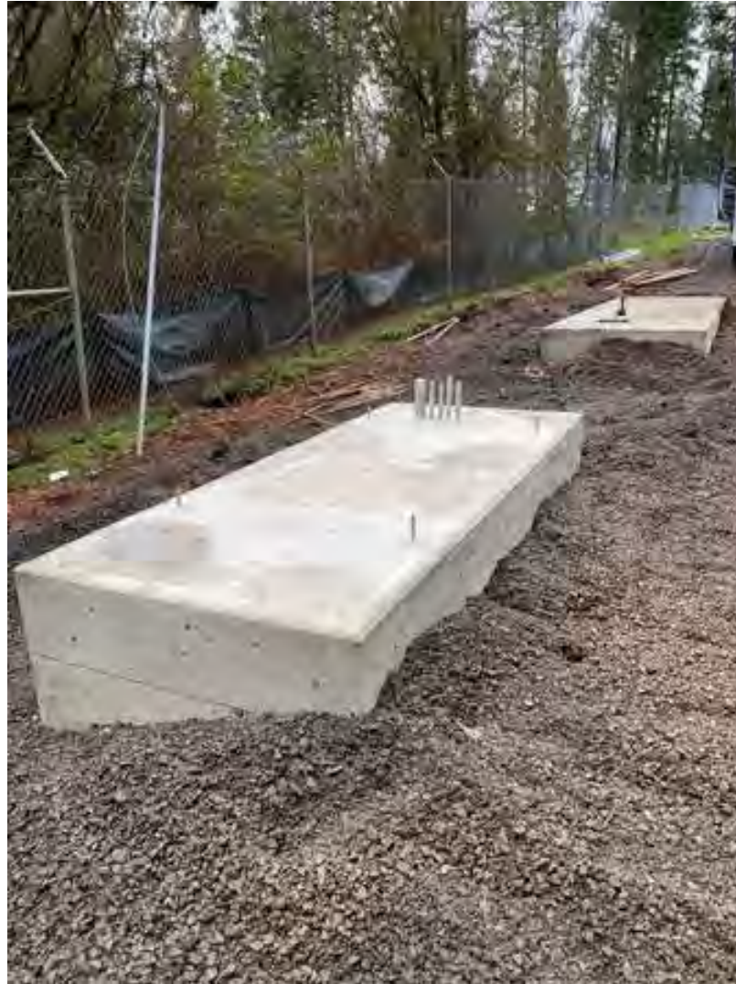
Wilsonville – Generator / Propane Slabs
